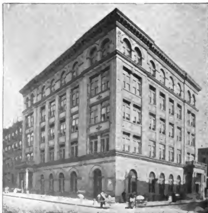
HEBREW INSTITUTE, EAST BROADWAY AND JEFFERSON STREET.
